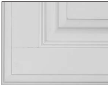
Example of front joint separation
