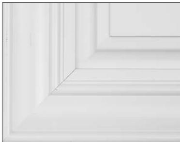
Example of front joint separation
