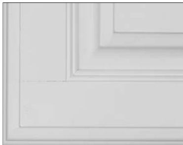
Example of front joint separation
