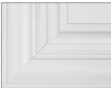
Example of front joint separation
